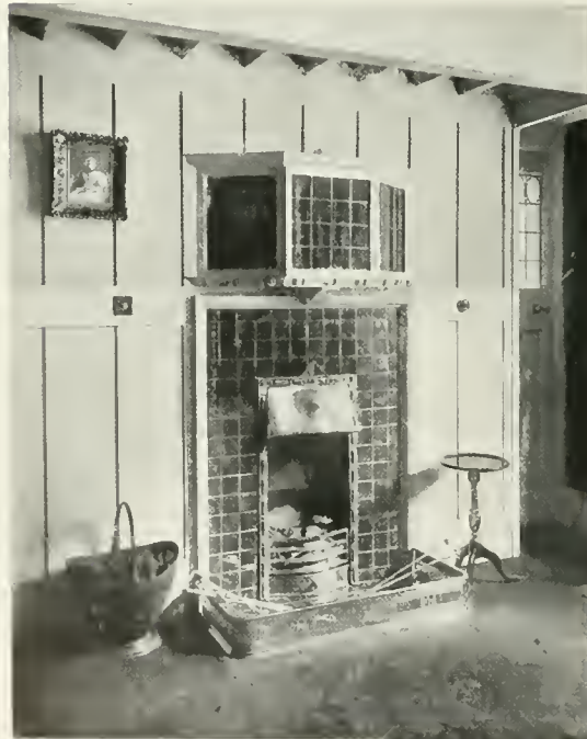
THE CHIMNEY CORNER IN A SITTING-ROOM, MARLBOROUGH CHAMBERS, JERMYN STREET, LONDON. SEE THE ILLUSTRATIONS ON PAGES 36 AND 37
